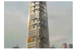
Gate Tower, Sharjah, UAE (Marley)
