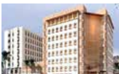
National Hospital Riyadh, KSA (Wefatherm)
