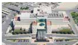
Saudi German Hospital Dammam, KSA (Wefatherm)
