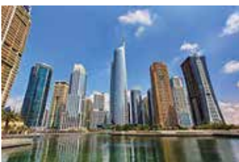
DMCC, UAE (Friatec)
