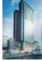
Crowne Plaza Dubai Marina, Dubai, UAE (Sanit)
