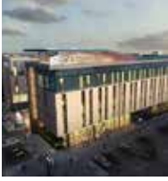
Aloft Hotel Garhoud, Dubai, UAE (dBlue & HDPE)
