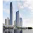
The Address Harbor Point, Dubai Creek, UAE (HDPE & dBlue)
