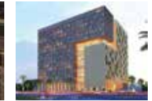
Hilton Garden Inn Hotel & Doubletree Suites, KSA (Wefatherm)
