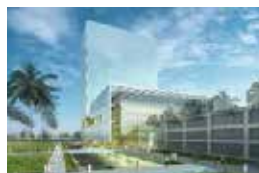
King Faisal Specialist Hospital & Research Center, KSA (Wefatherm)
