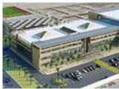
American International School Jeddah, KSA (Wefatherm)
