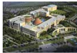
RIT University Campus, Dubai, UAE (Wefatherm, HDPE, dBlue & Sanit)
