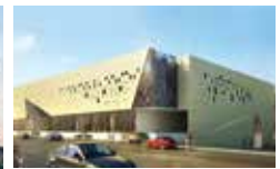
Emirates Hospital Mirdif, Dubai, UAE (Wefatherm)
