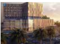
King's College Hospital, Dubai, UAE (dBlue & HDPE)
