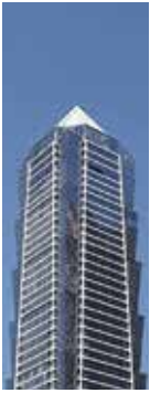
Al Batha Tower, Business Bay, UAE (Marley)
