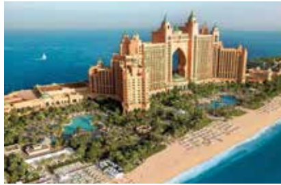
Atlantis Hotel, Water Line Maintenance, UAE
