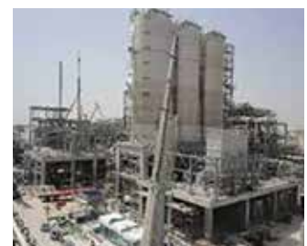
Revamping of WWTP in Ethylene Plant, Qatar
