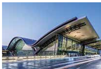
New Acid Line at Hamad International Airport, Qatar
