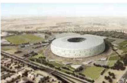
Al Thumama Stadium, Qatar
