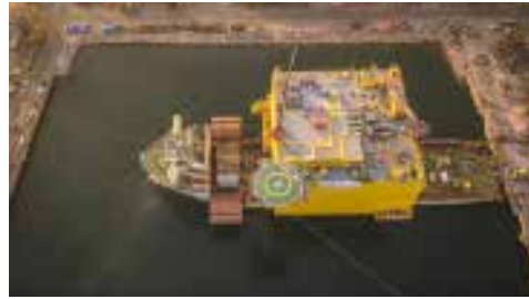
BorWin-3 - Fire Fighting Network Repair, UAE
