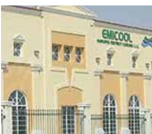
Emirates District Cooling EMICOOL Dubai, UAE
