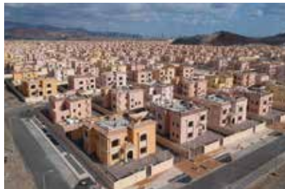
Water Network & House Connections - MBZ City in Fujairah 1100 Housing Units, UAE
