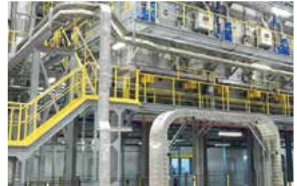
Ma'aden - Civil Works Project, KSA
