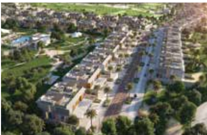
Dubai Hills Estate (LPG Plant & Network), UAE
