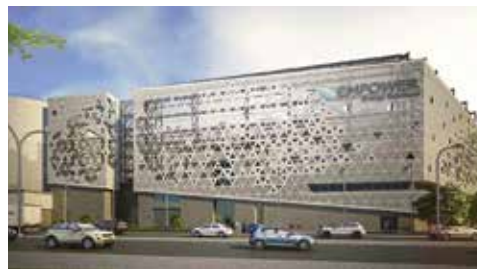
Jumeirah Village Circle JVC District Cooling Plant, UAE
