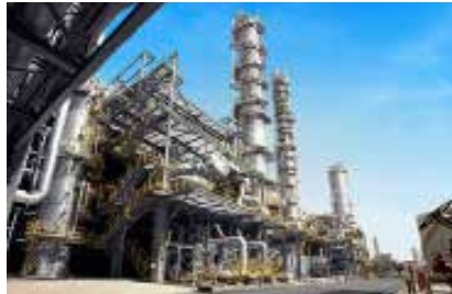
Upgrade Firefighting Network at Safaniyah Petrochemical Plant, KSA
