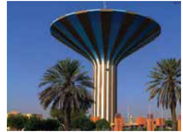
Riyadh Water Tower Refurbishment, KSA
