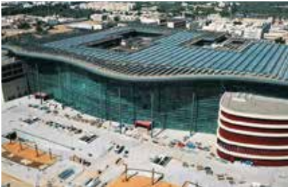
Water Connections to the New Al Ain Hospital at Al Mutaredh, UAE
