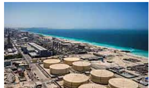
Jubail phase IV potable water plant, KSA
