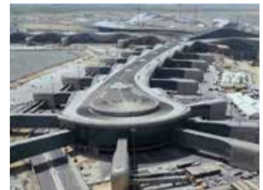
Abu Dhabi Airport, UAE
