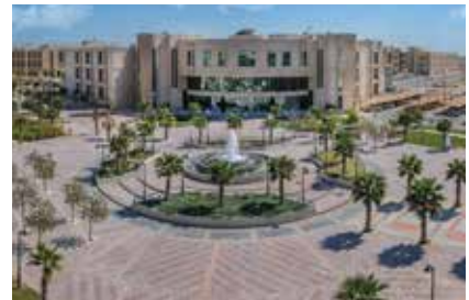
Gas Network Dammam University, KSA
