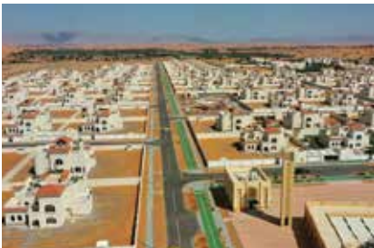
Water Services - Emirati Housing Project Al Hayer, UAE
